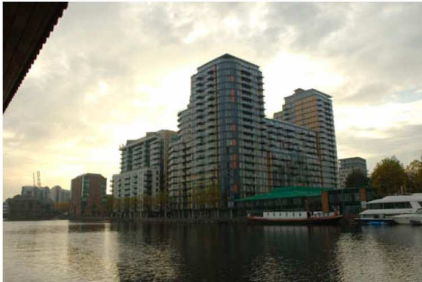
Existing View from North-East of Building
